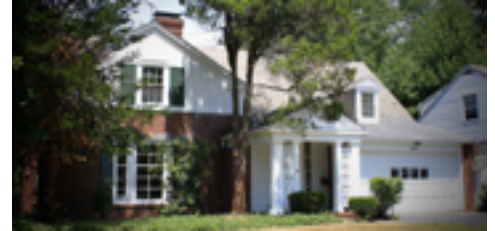
NEW! 3393 HOLLISTER ROAD RENOVATION COMPLETED SEPTEMBER 2009
