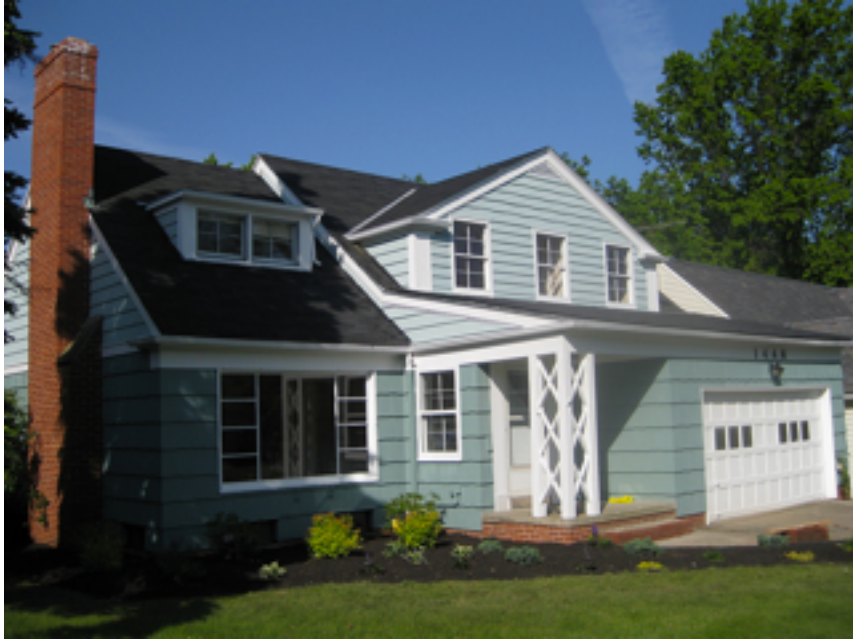
1446 WESTOVER ROAD RENOVATION COMPLETED MAY 2010
