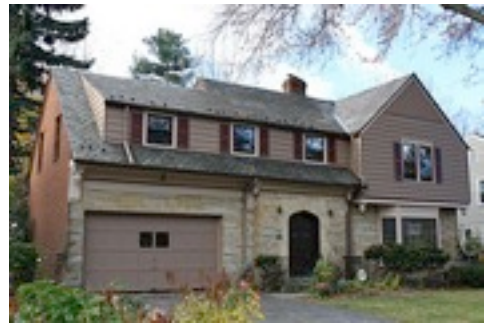
1420 BLACKMORE ROAD RENOVATION COMPLETED DECEMBER 2009
